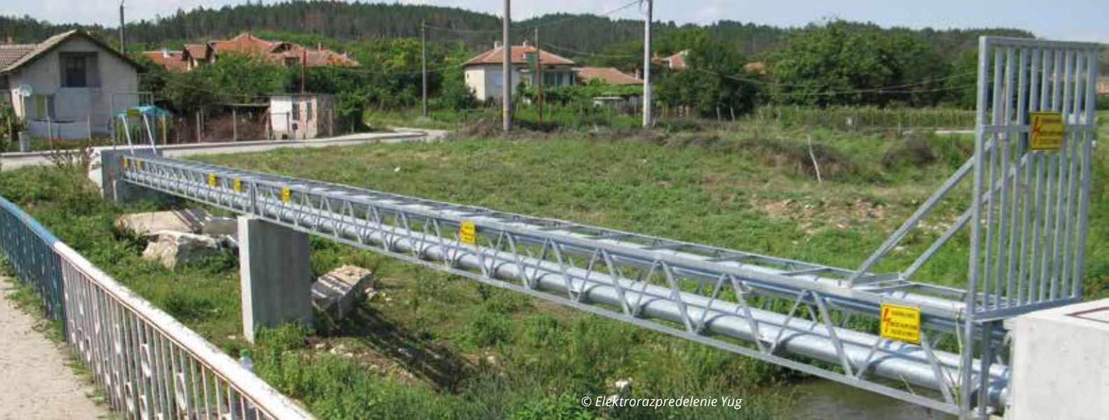
Specialized safety feature – the so called “Catwalk Bridge” for the carriage of underground cables over a river
