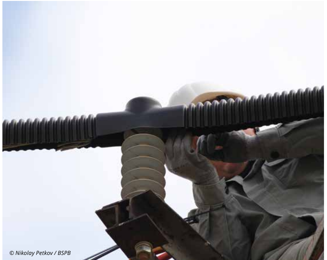
Installation of protective insulations on poles
