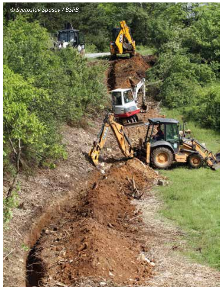
A trench for laying of underground power lines
