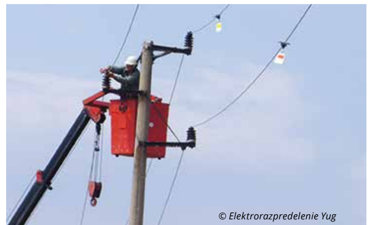
Installation of diverters under the “Life for the Burgas Lakes” project
