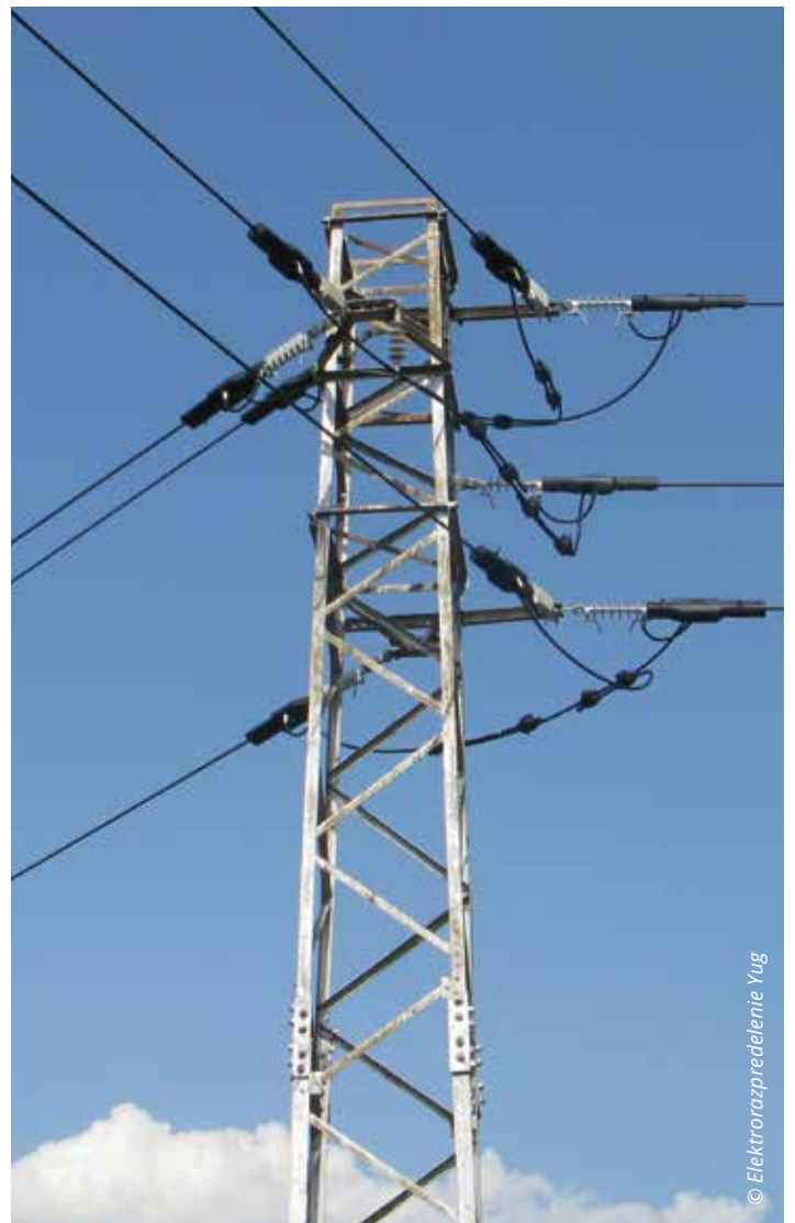
Shielded pole with a PAS system (a system of insulated conductors)
