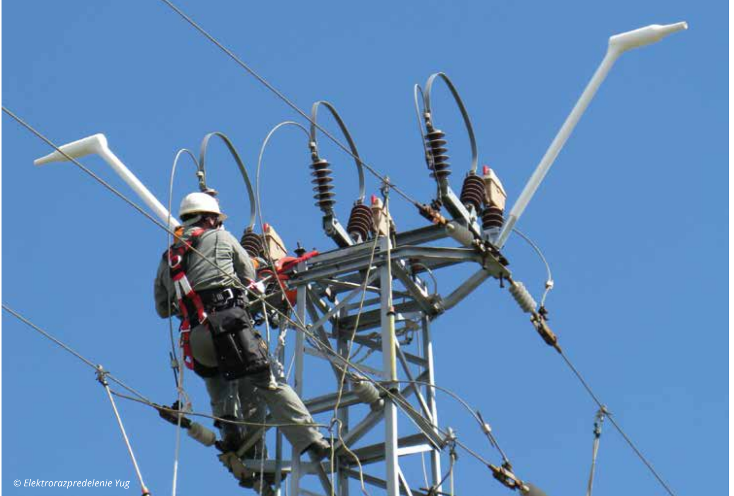
Installation of birds rests by Elektrorazpredelenie Yug
