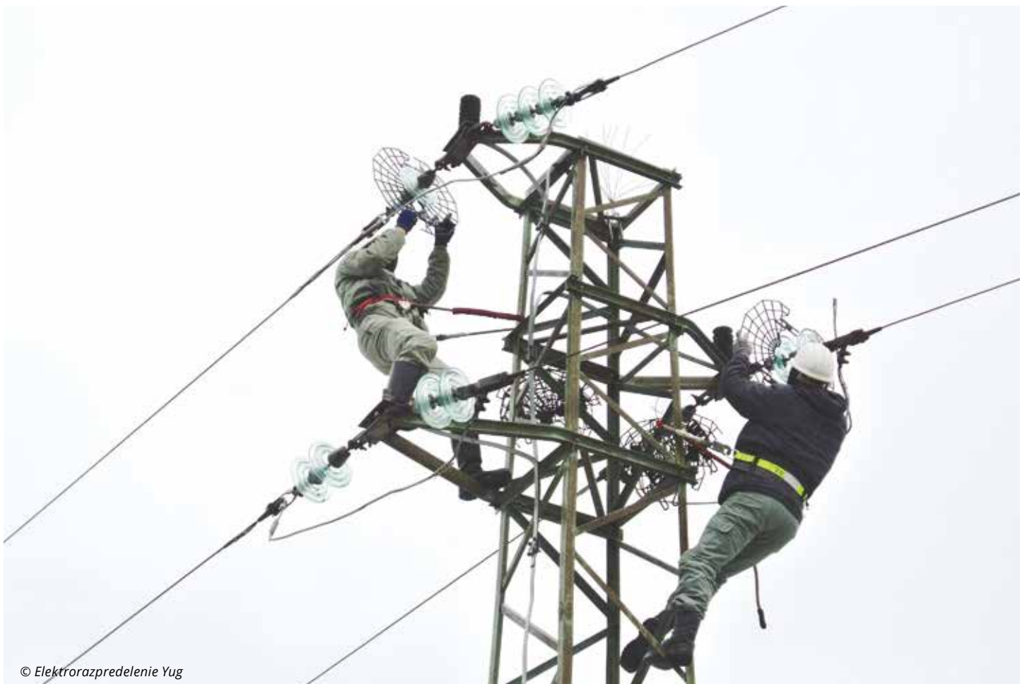
Installation of protective plastic gratings for birds on poles from overhead power lines
